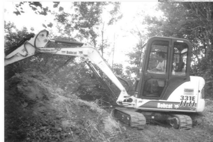
Ed French excavates a trench for the dredge discharge pipe
